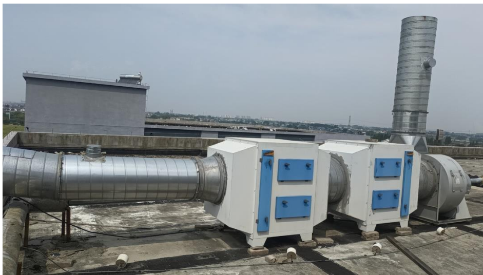
废气收集管道和集气罩
