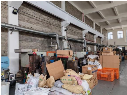
废气收集管道和集气罩
